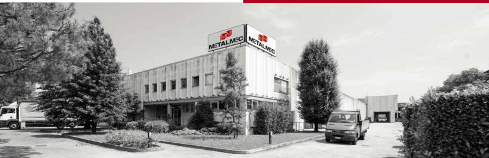
The large headquarters at Mapello (BG), Italy, with over 4000 sqm dedicated to production and warehouses.
